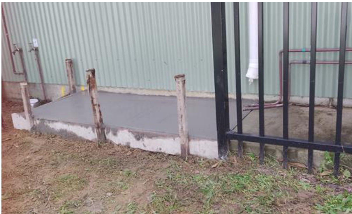
Cement slab for dust extractor.
